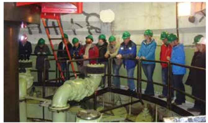
Tour group looking down into one of the turbine generating units at the Mactaquac Dam. October 22, 2015.
