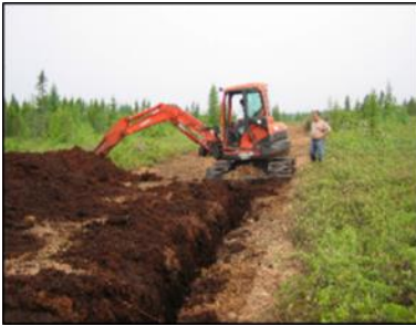
Figure 1a – Excavating a peripheral ditch
